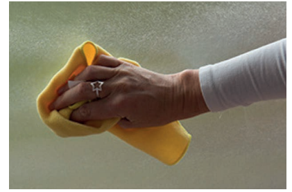
Dry surface with a cloth, leave to dry completely (takes around 48 hours).
