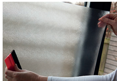
Apply onto the glass and slide the vinyl into place leaving a gap away from the edge. Use a d-c-fix smoother or squeegee to remove any excess water.
